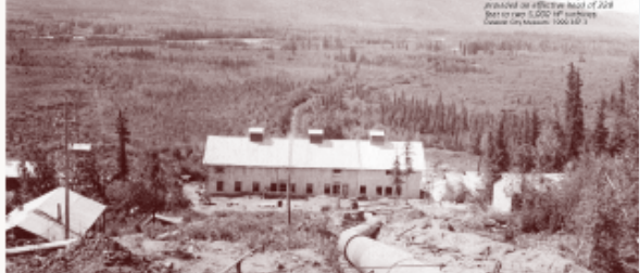
North Klondike Power House, completed in 1911. The power house was a 1000-horsepower plant, which was the largest in the Klondike region. It was built by the Klondike River Hydroelectric Plant, which was the first power plant in Yukon. The power house was built on the Klondike River, a site that would be 20 miles that served in a very different way. Generators were provided for a few years in the morning. The rates were clearly indicated on the meter used by the consumers and reached 10 cents by the end of the second World War.
